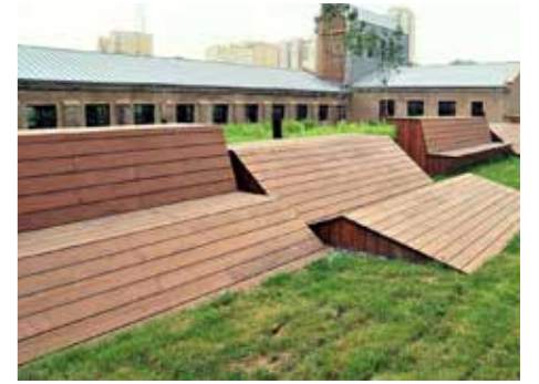
Reconstruction of Jilin Waterworks
